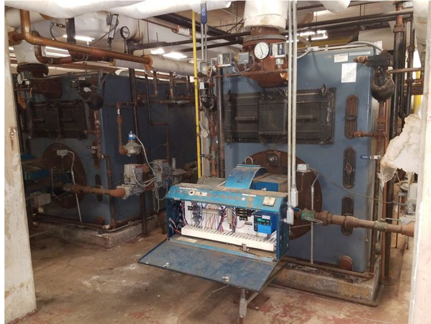
Dows Lane Boiler - Failing pipes and sessions
